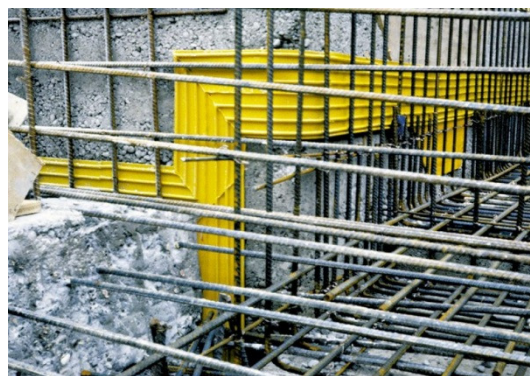
Figure 11: Rebar and Water Bar Installation
