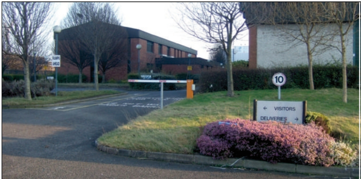
Photo 1: Uniphar Office Building 1
