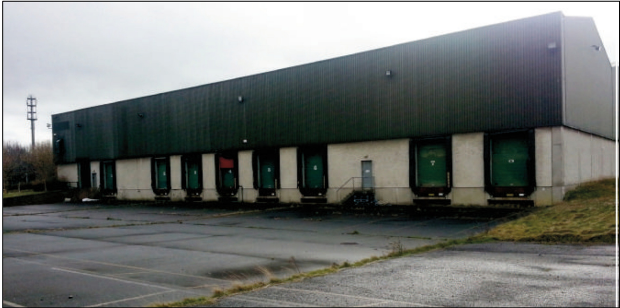
Photo 2: Uniphar Warehouse – Building 2
